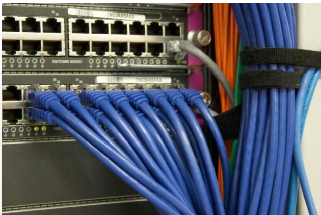
Data Cables terminated on Ethernet Switch
